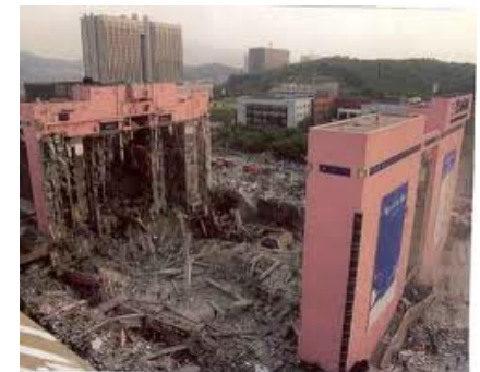
• Department Store Collapse
